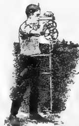
Trimming Side of Hedge
